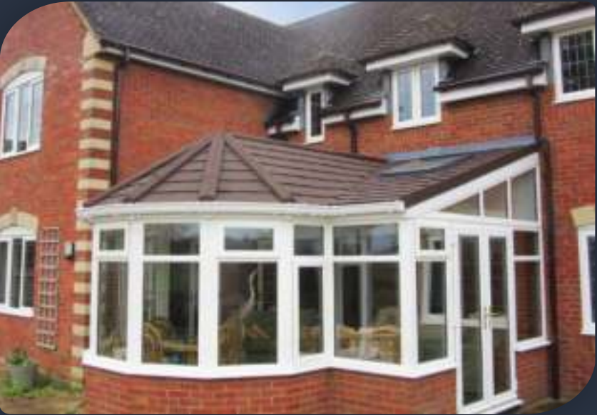
Combination extension layout, with Icotiles and Velux.
